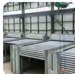
Hoisting area Horizontal structure
