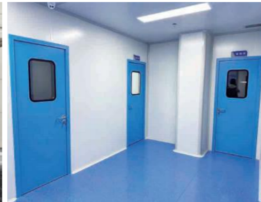
Steel swing door of the purification workshop
