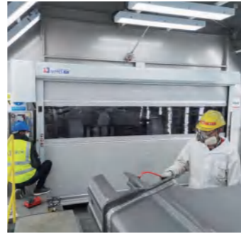
Painting equipment room
